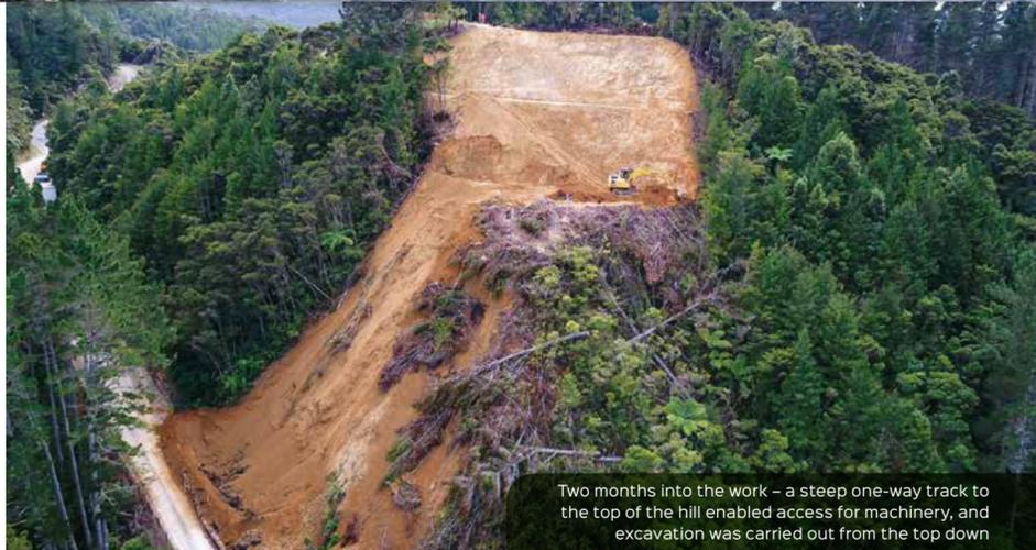
Two months into the work – a steep one-way track to the top of the hill enabled access for machinery, and excavation was carried out from the top down
